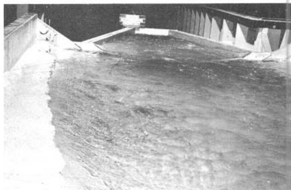
A. Somewhat turbulent water surfaces occur in the transition and canal. Q=4.7 c.f.s., V_p=6.0 f.p.s., canal depth=1.3 D.
