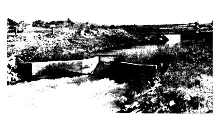
Figure 4.—Four-foot Parshall flume discharging 62 ft³/s (1.76 m³/s) under free-flow conditions. Scour protection is required with this height of fall. (Courtesy U.S. Bureau of Reclamation.)
