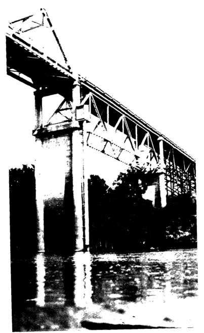
FIGURE 28.—Corrugated-steel-pipe well and wooden shelter attached to bridge pier.
