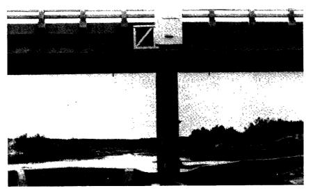
FIGURE 7.—Artificial control on Delaware River near Red Bluff, New Mex., with shallow V notch in the broad-crested weir.
