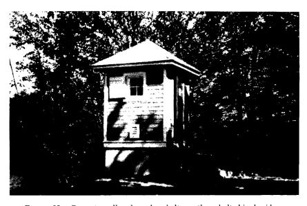
FIGURE 23.—Concrete well and wooden shelter with asphalt-shingle siding.
