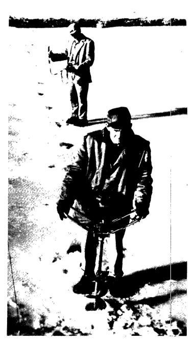
FIGURE 93.—Ice rod being used to support current meter for a discharge measurement, top; ice drill being used to cut holes, bottom.
