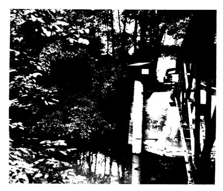
FIGURE 27.—Steel-pipe well and look-in shelter attached to bridge abutment.
