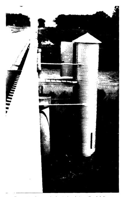
FIGURE 24.—Corrugated-galvanized-steel-pipe well and shelter.
