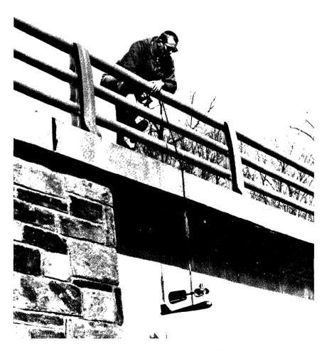
FIGURE 62.—Handline in use from a bridge.
