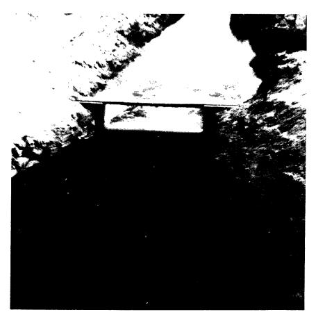
FIGURE 3.—Rectangular weir on Trifolium Drain 23 of Imperial Irrigation District, near Westmorland, Calif. (View looking downstream.)
