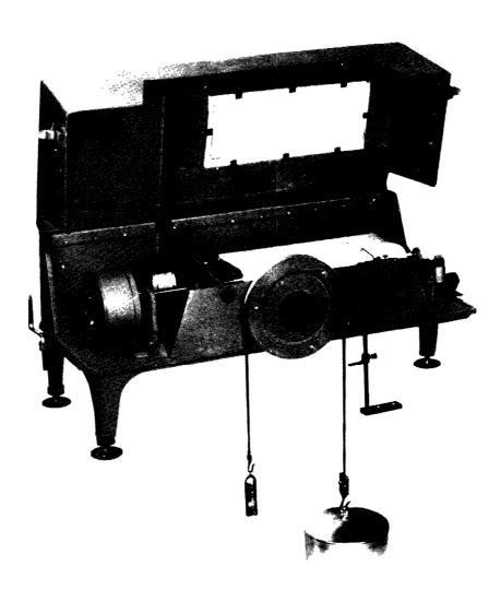
FIGURE 19.—Continuous strip-chart recorder.
