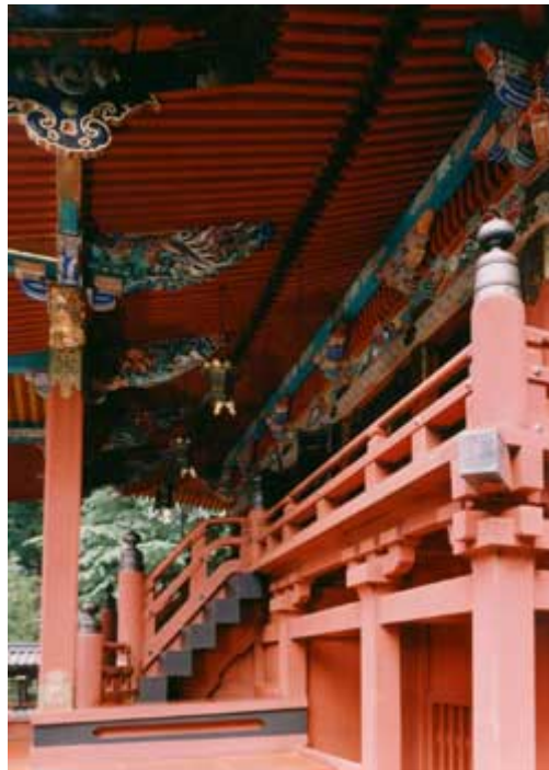
Figure 8. The Honden, the main hall of Futarasan-jinja (mainly constructed from wood) ( http://www.city.nikko.lg.jp/kankou/shaji/english/main.htm )
