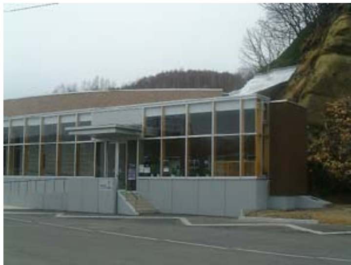
Figure 2. The old and new office building of the Fugoppe Cave ( http://www.amateras.com/trip/japan/hokkaido/otaru-e.htm )
