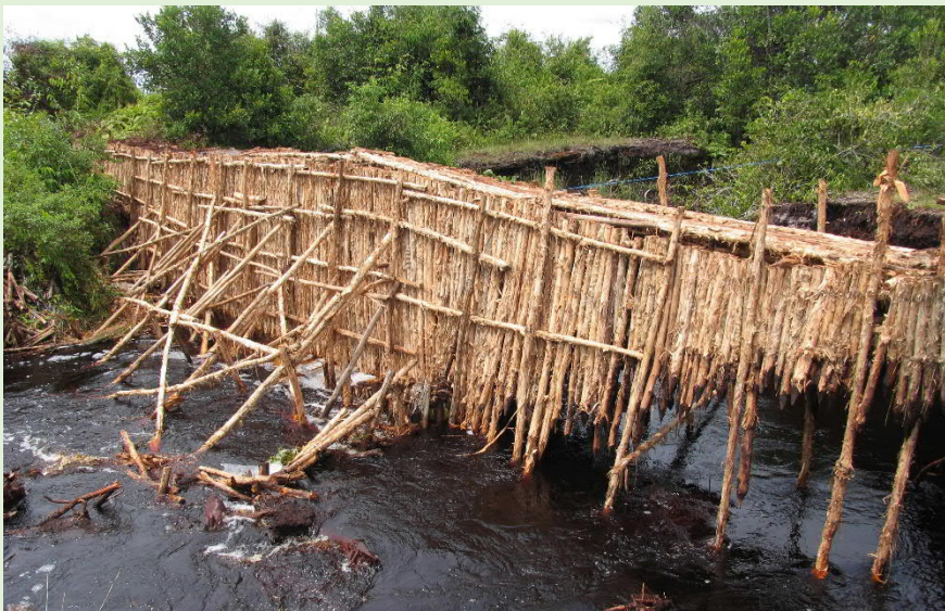
A lesson from the early RESTORPEAT dams: because the gelam poles did not extend into the mineral subsoil, the dam was subsequently undermined by seepage and collapsed.
