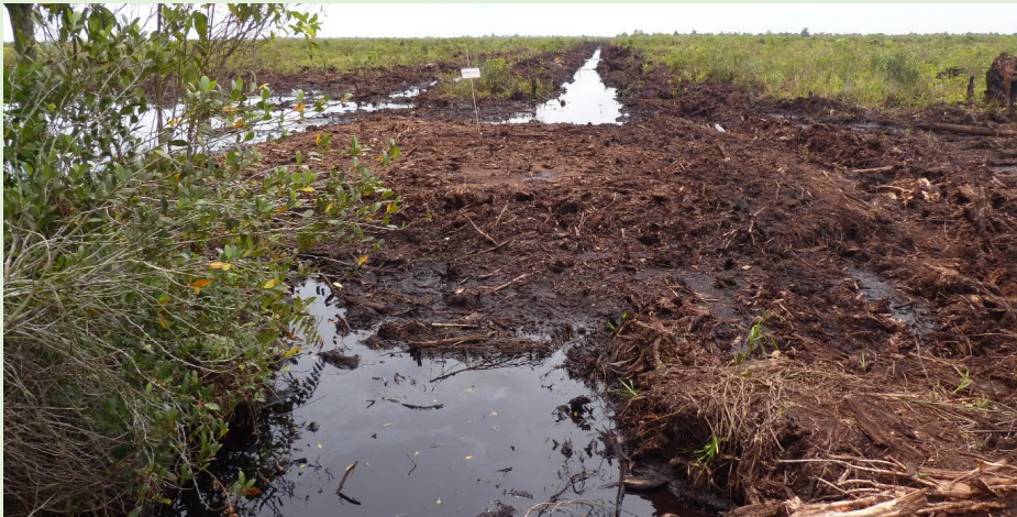
Compacted peat block over a 2-3m wide canal
