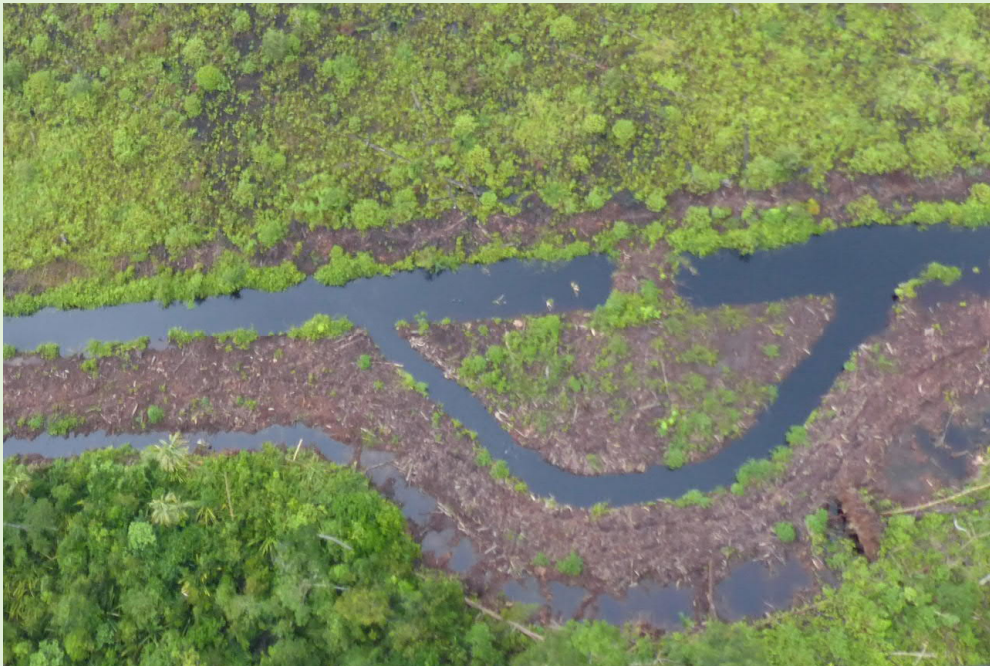
Aerial view of a compacted peat dam with a lateral spillway or bypass (at -50cm), in one of the APP related concessions in South Sumatra. In full rewetting a bypass is not desirable.
