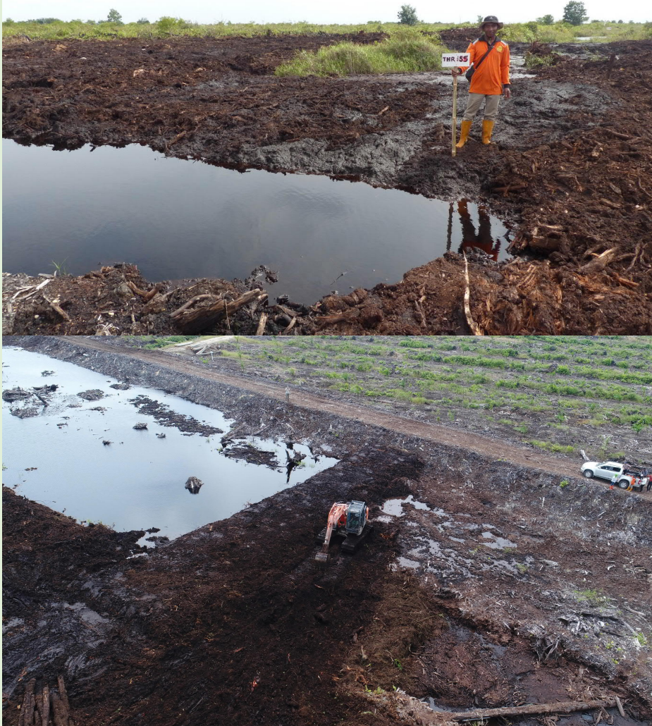
Compacted peat block over an 8m wide canal
