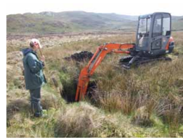
First suite of Pumlumon Project ditch blocking works being carried out on private farm land by a local contractor © MWT
