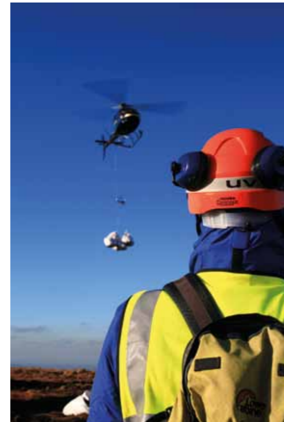
Marshalling bags of heather brash on to bare peat © Moors for the Future Partnership
