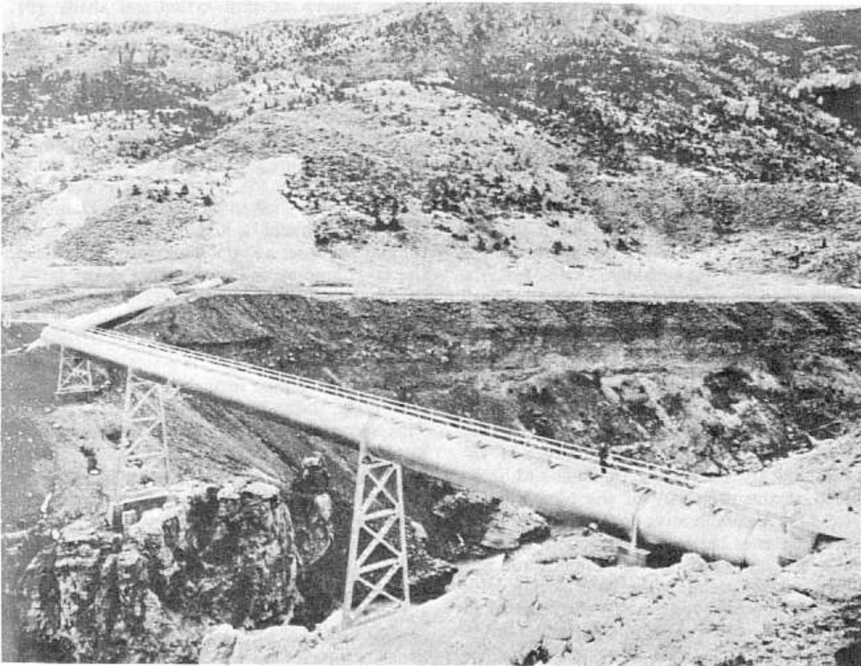
FIGURE 16.—The Shoshone River siphon crosses the river on a 150-foot span.
