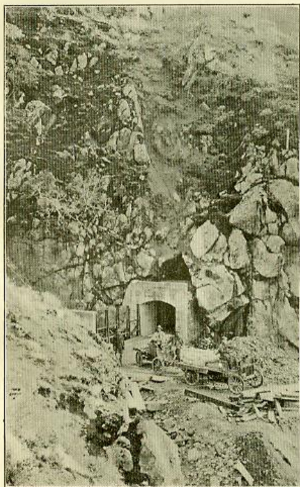
FIG. 170.—Flume between Tunnel Portals, Southern California Edison Co.
