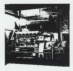
34 Fully-automatic emergency Dieselgenerator set for a pumping station.
