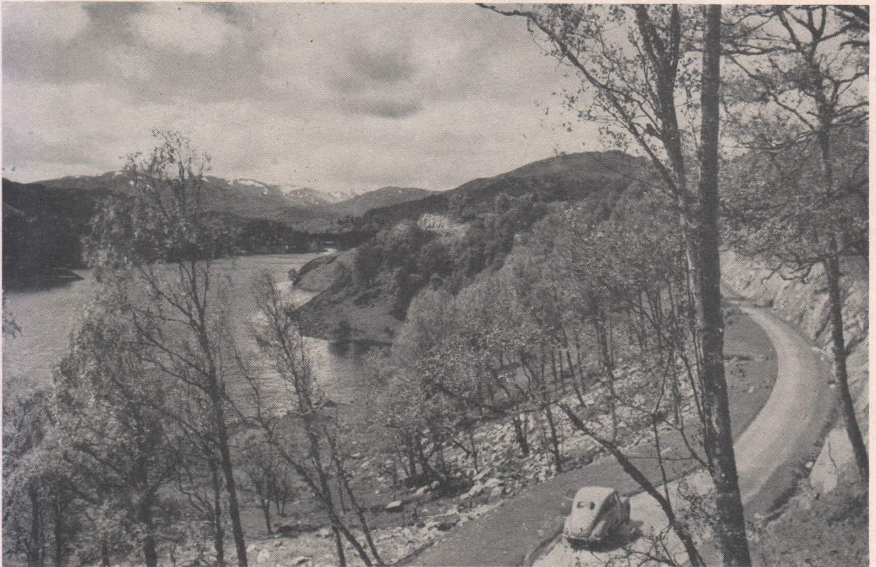
Fig. 1. Loch Benevean at the new level, showing part of the road diversion to Glen Affric
