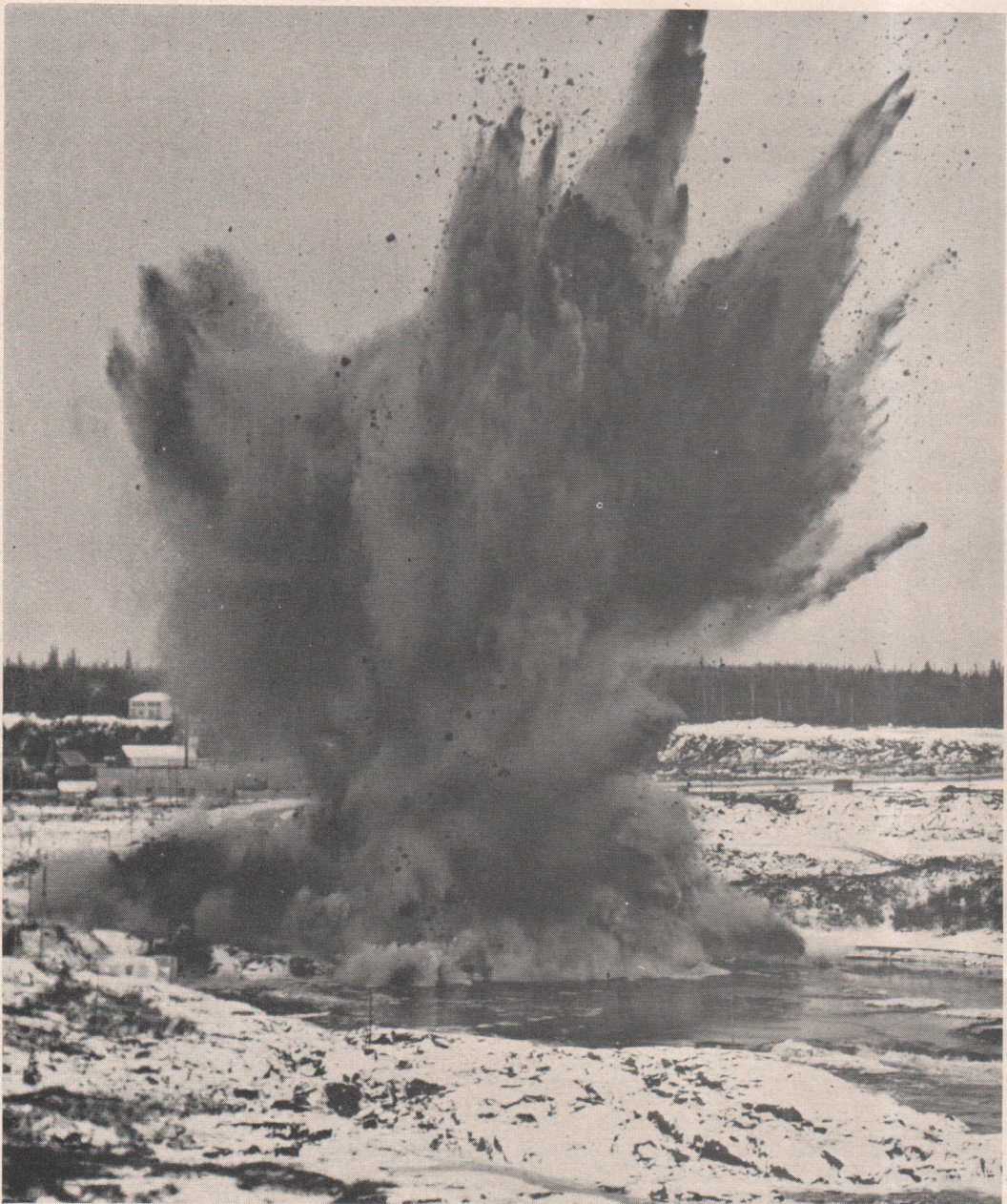
Fig. 1. Blasting the downstream rock plug of the diversion tunnel
