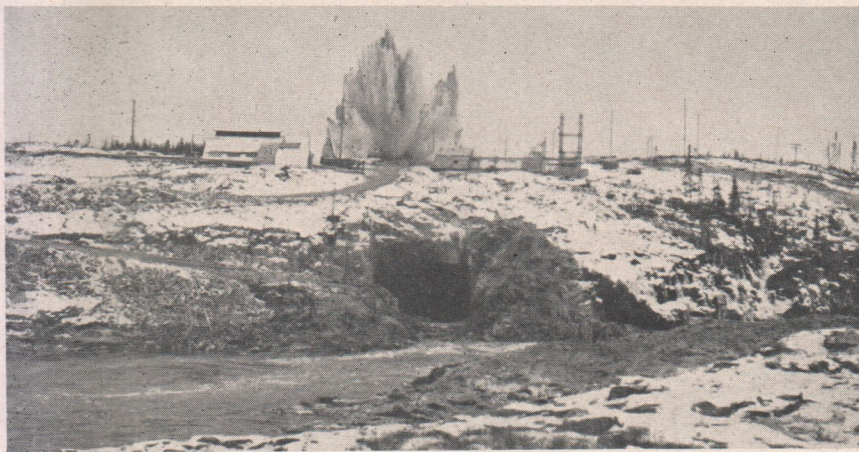
Fig. 2. Downstream tunnel mouth and upstream plug being blasted
