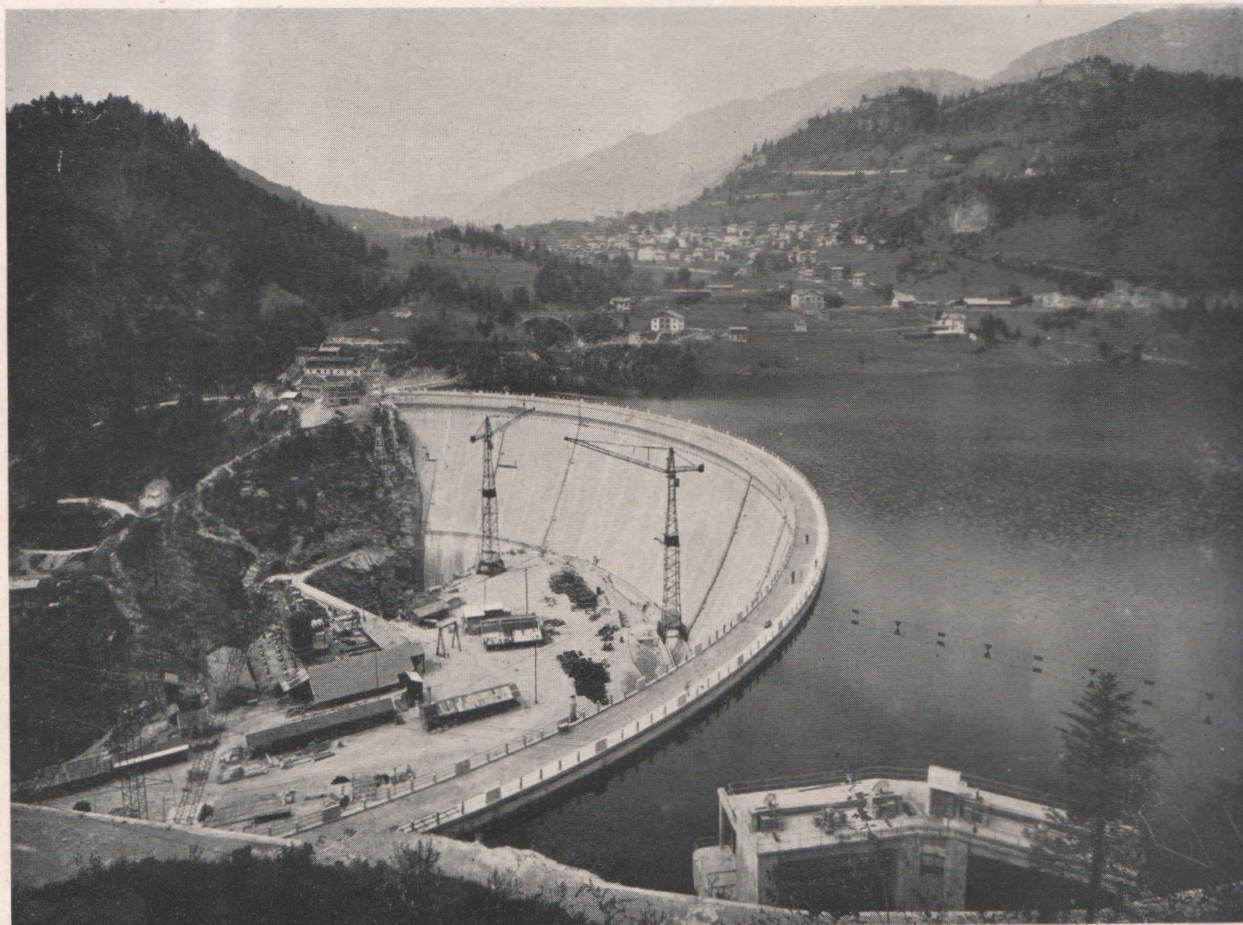
Fig. 1. General view of the Pieve di Cadore dam
