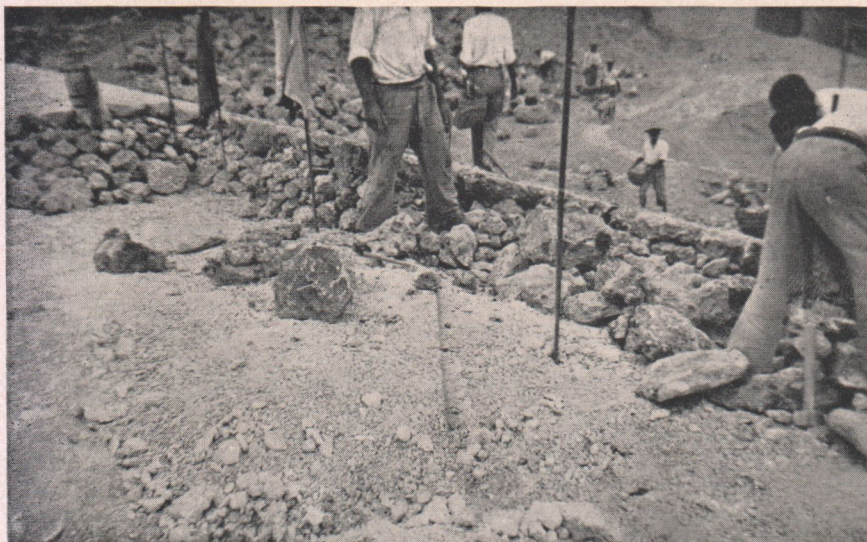
Fig. 6. Filter construction at Cubillas
