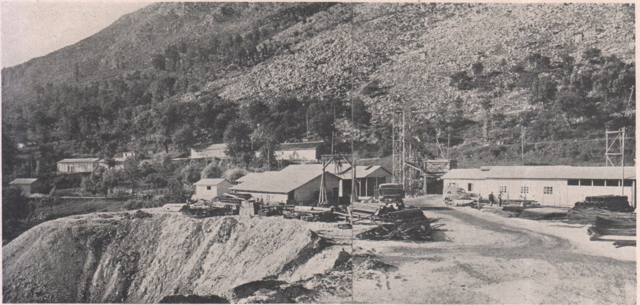
Fig. 1. View of the works at the Venafro end of the tunnel
