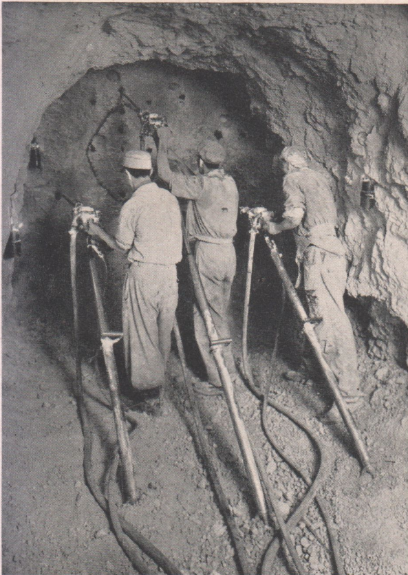
Fig. 7. Three Atlas RH 655W drills at work in the pilot tunnel
