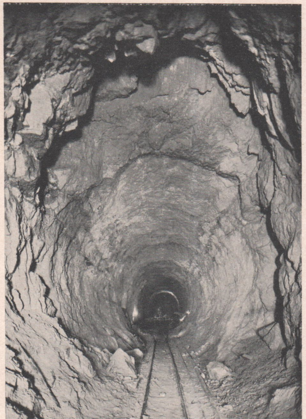
Fig. 8. A portion of the Rocca d'Evandro tunnel before being lined
