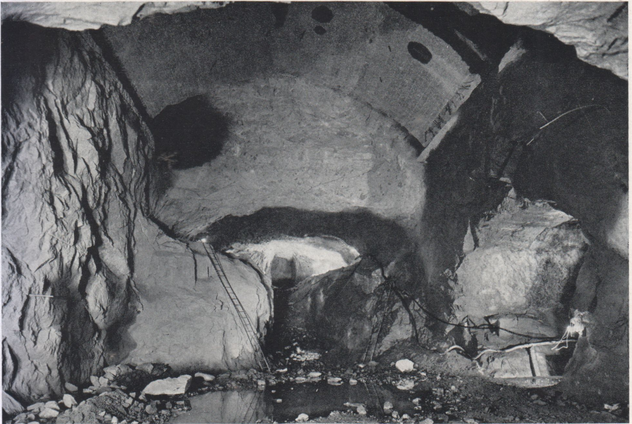
Fig. 57. Malga Boazzo machine hall being excavated in granodiorite
