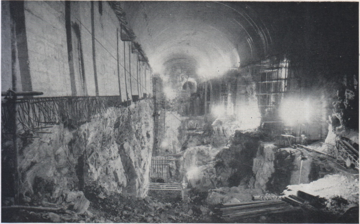
Fig. 55. Kariba machine hall under construction in gneiss
