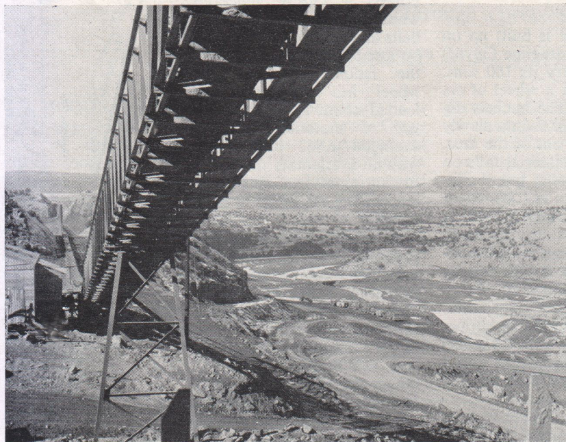
Fig. 5. Main conveyor belt seen from loading station
