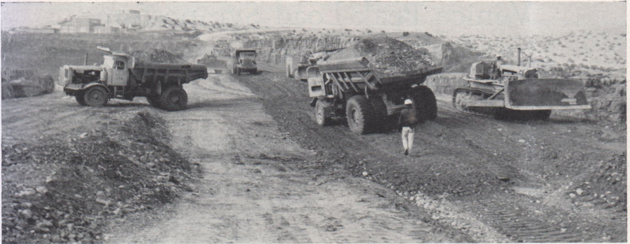
Fig. 8. A view of work on the embankment
